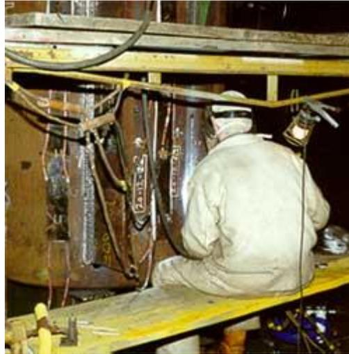
Preheating of a jacket structure to prevent hydrogen cracking
